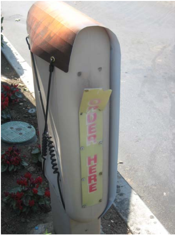
ORDER HERE sign needing to be replaced
